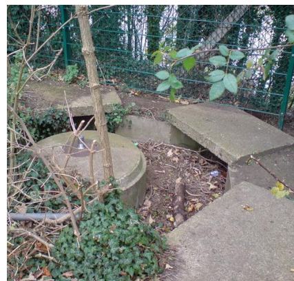
Fixed Spigot mortar point
